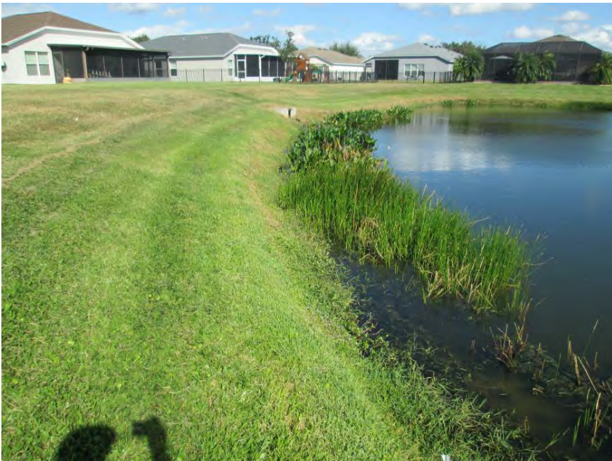
Pond 35 – north bank +/-18” vertical drop, viewing east
