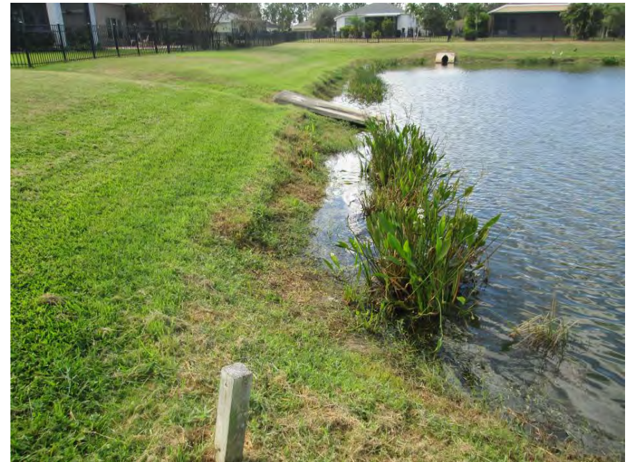
Pond 35 – south bank +/-18" vertical drop, viewing west
