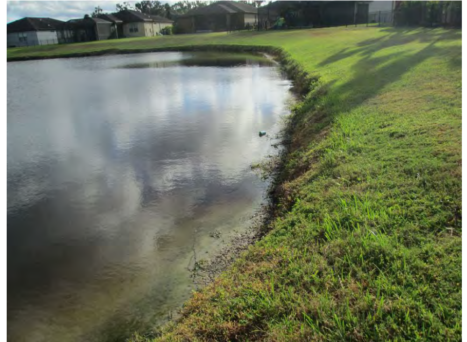
Pond 17 – north bank viewing west 18"-24" vertical drop
