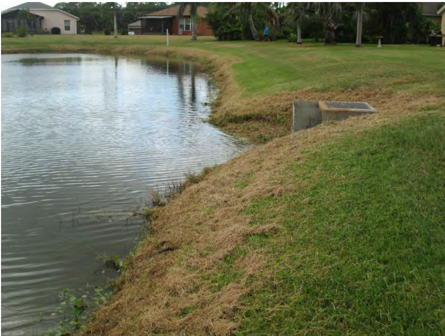
Pond 34 – Control Structure inset in north bank
