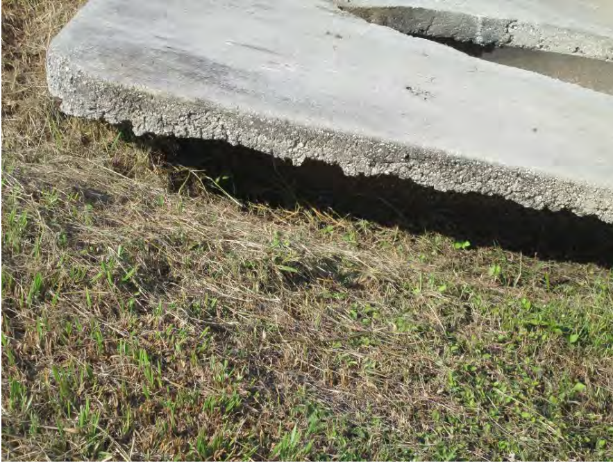
Pond 35 – MES on south bank undermined and eroded
