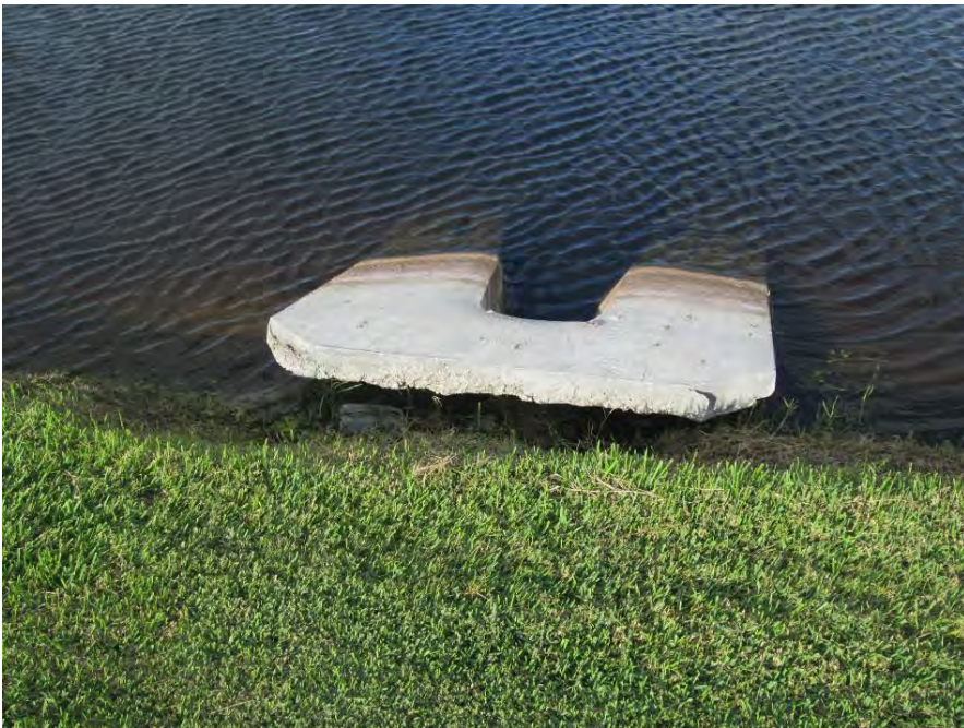
Pond 17 - Undermined & eroded MES on west bank
