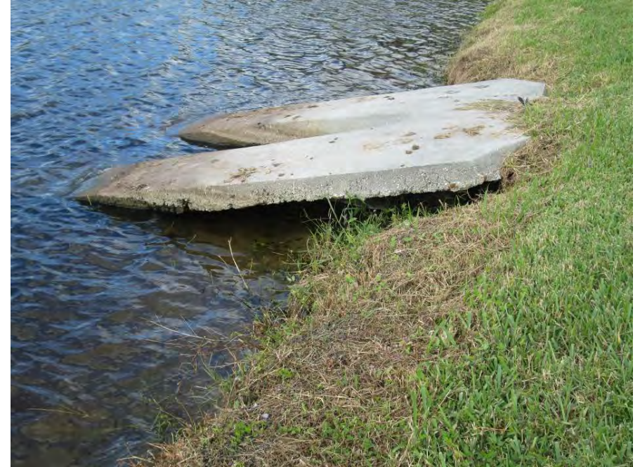
Pond 17 - Undermined & eroded MES on south bank
