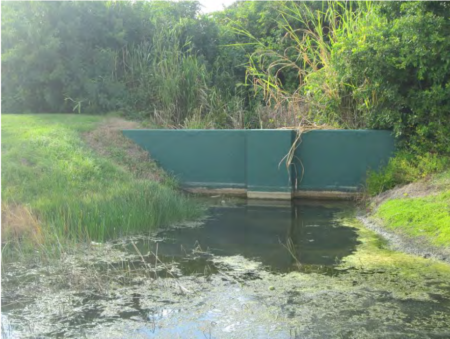
Pond 19 – Outfall weir on west side
