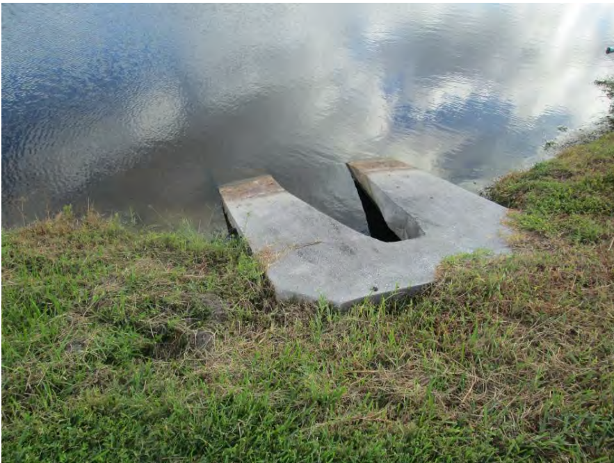
Pond 17 – Undermined and eroded MES on northeast corner
