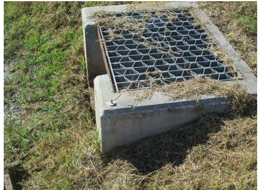
Pond 35 – Control Structure on north bank, no skimmer, large opening
