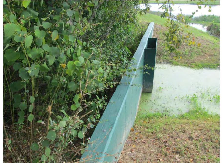
Pond 37 – Outfall weir on northeast portion of pond, cut back vegetation 10'
