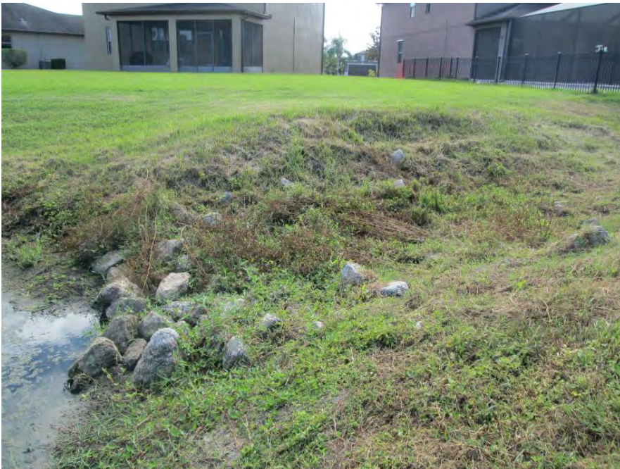
Pond 29 – swale on northwest portion of pond, steep banks
