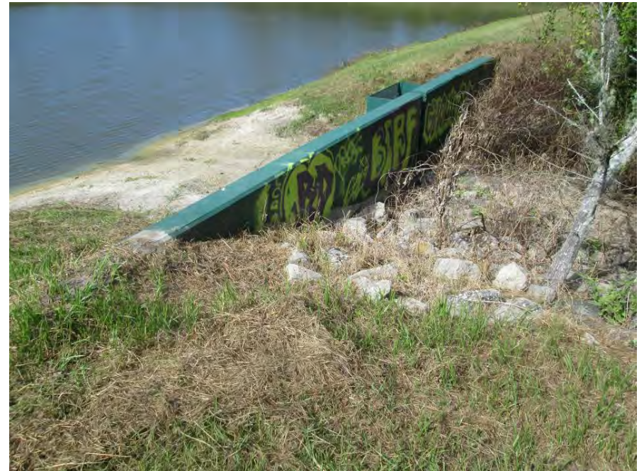
Pond 29 – Outfall weir on east side of pond
