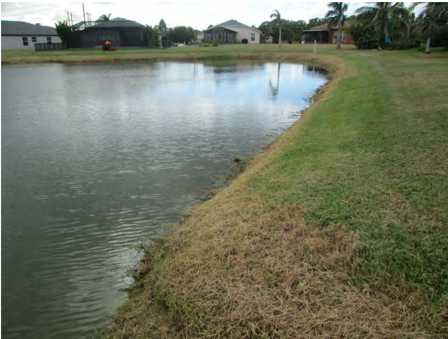
Pond 34 – north bank viewing west +/- 18” vertical drop
