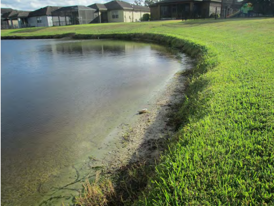
Pond 17 – north bank viewing west 18”-24” vertical drop
