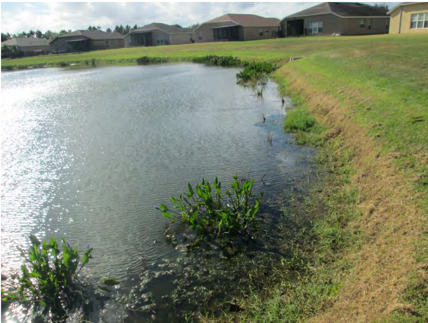
Pond 35 – north bank +/-18" vertical drop, viewing west
