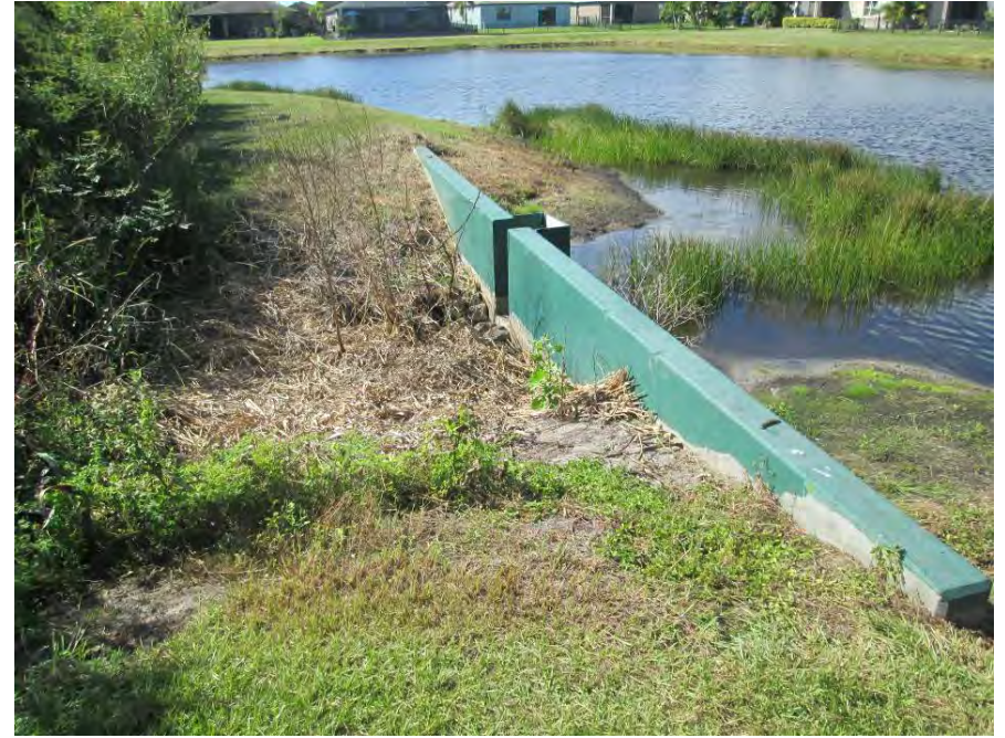
Pond 30 – Outfall weir on south side
