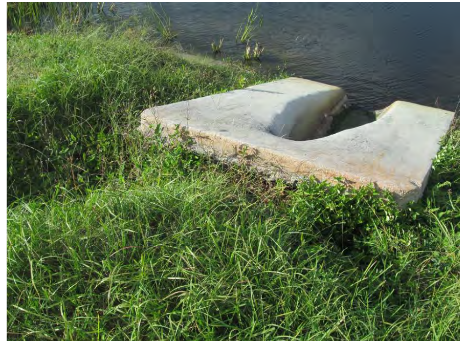
Pond 19 – MES Undermined and eroded
