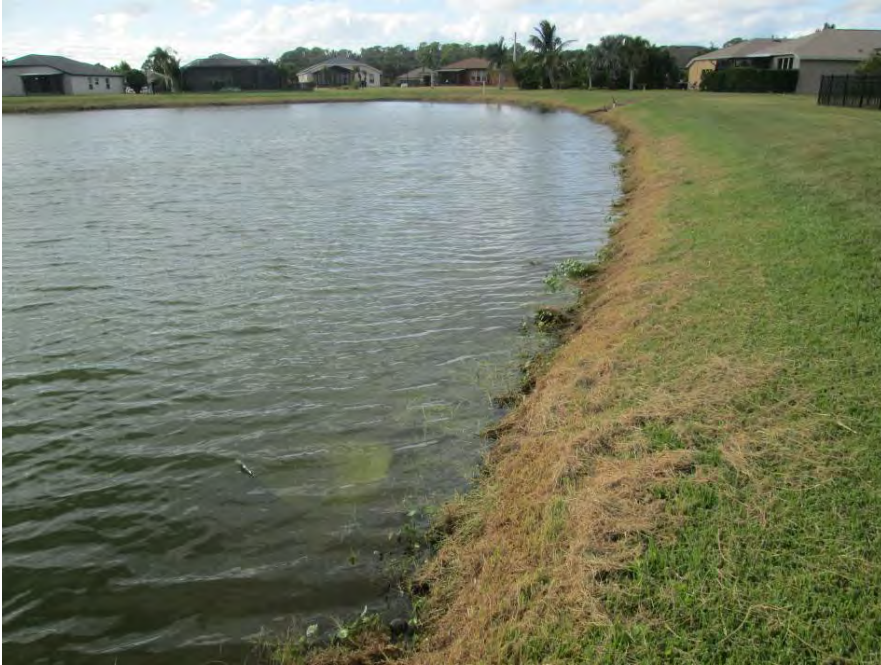
Pond 34 – north bank viewing west +/- 18” vertical drop
