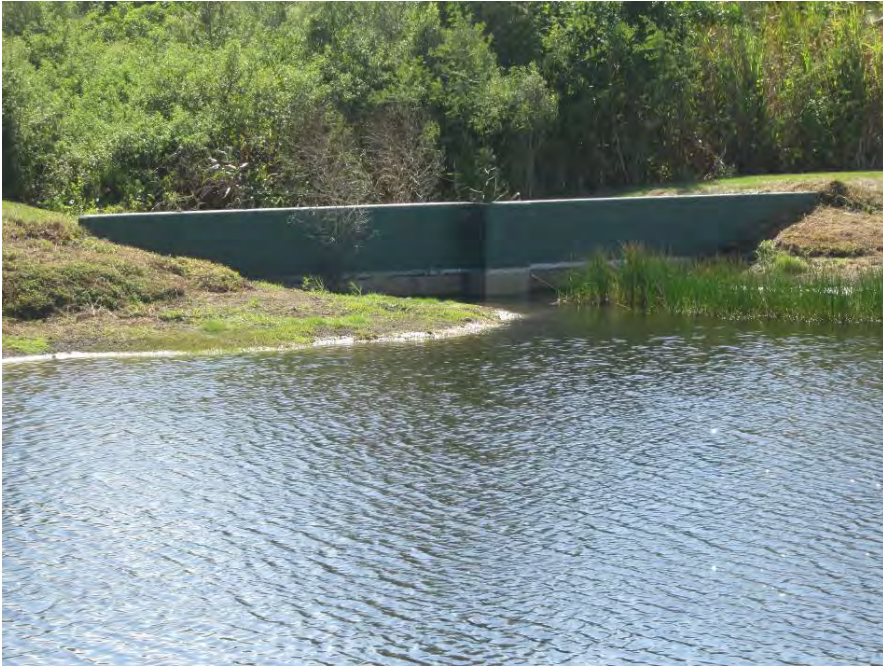
Pond 30 – Outfall weir on south side
