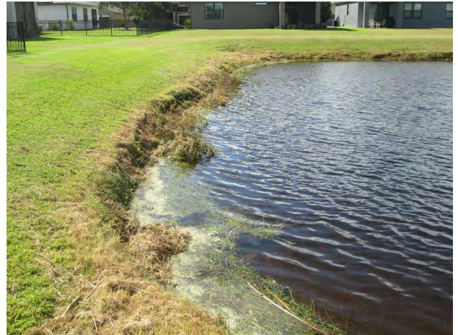
Pond 32 – south bank viewing west 18" vertical drop
