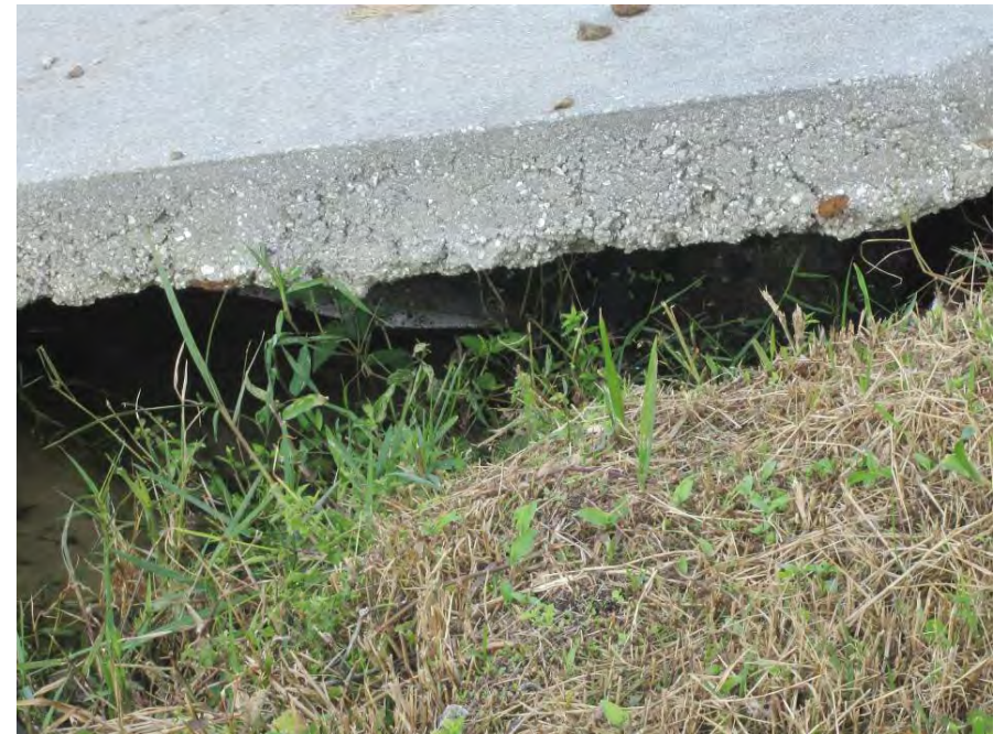
Pond 17 - Undermined & eroded MES on south bank
