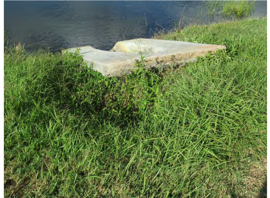
Pond 19 – MES Undermined and eroded
