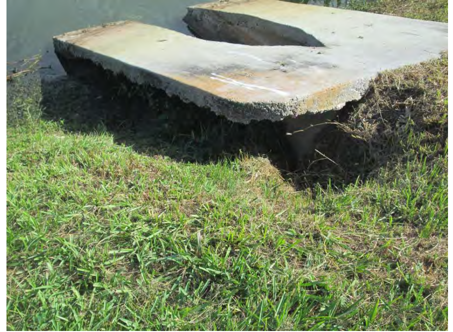
Pond 35 – MES on west bank undermined and eroded
