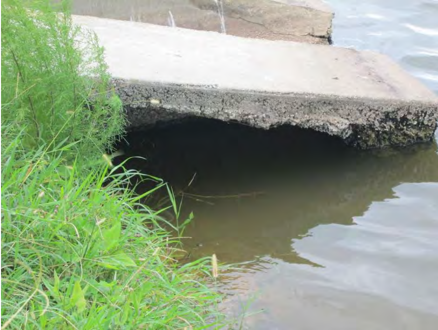
Pond 36 – MES on south bank undermined and eroded
