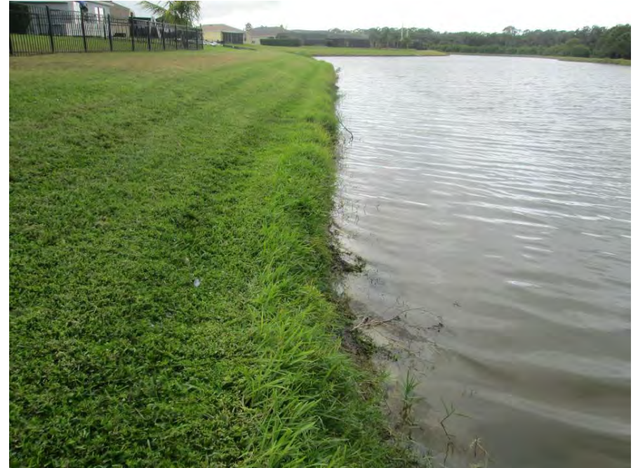
Pond 36 – south bank 18'' vertical drop, viewing west
