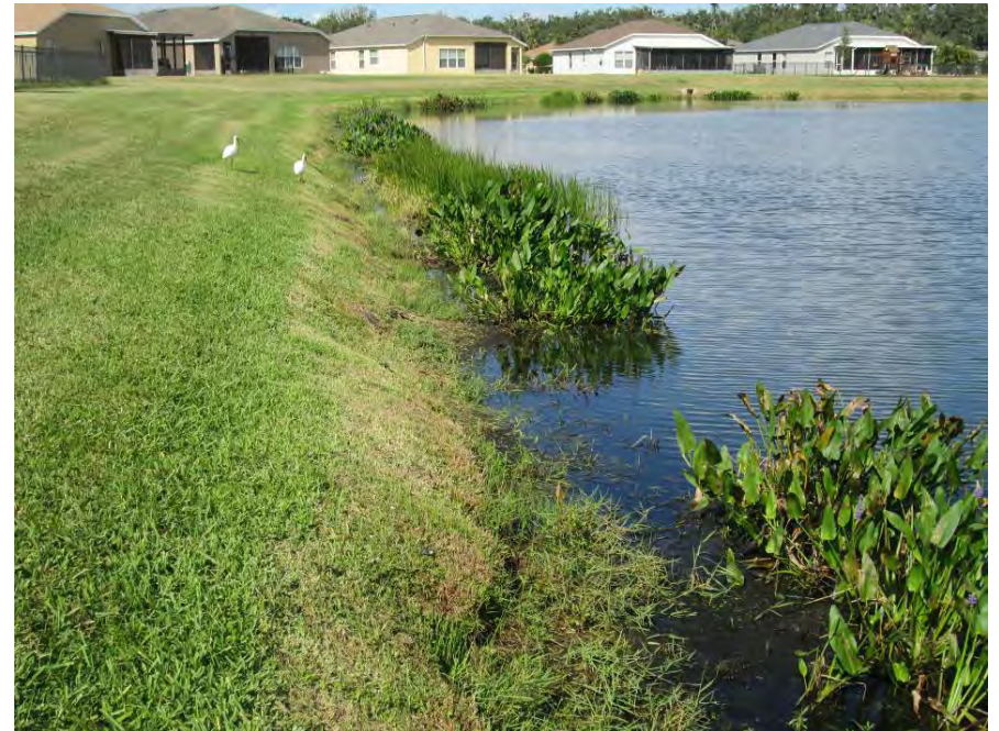
Pond 35 – west bank +/-18" vertical drop, viewing north
