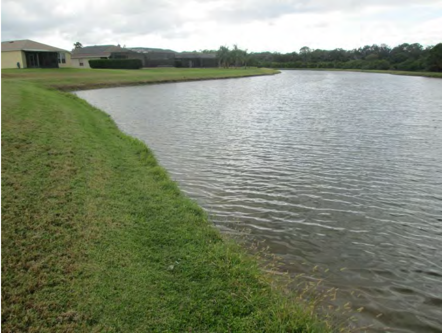
Pond 36 – south bank 12” vertical drop, viewing west
