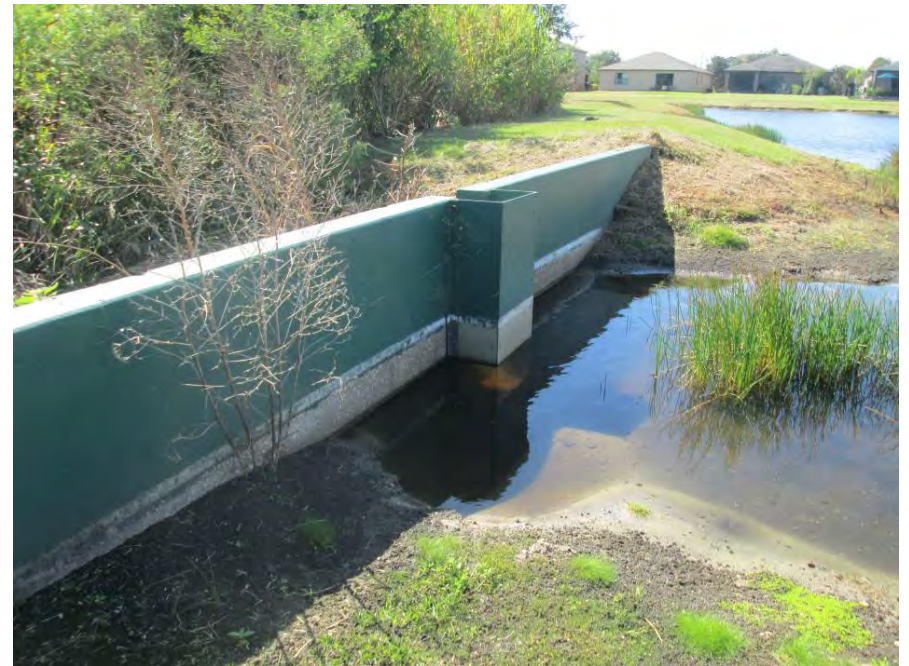
Pond 30 – Outfall weir on south side
