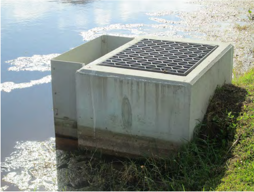
Pond 40 – Control Structure on north bank
