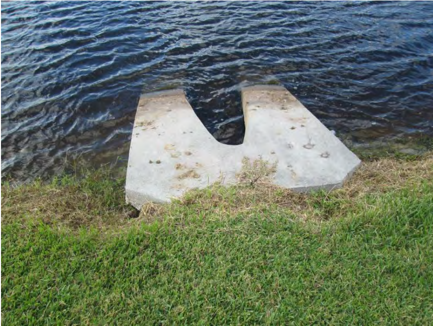
Pond 17 - Undermined & eroded MES on south bank
