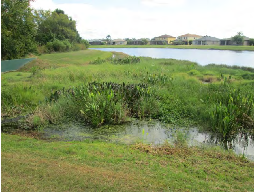
Pond 37 – littoral shelf on northeast portion of pond
