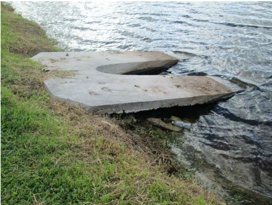
Pond 17 - Undermined & eroded MES on south bank
