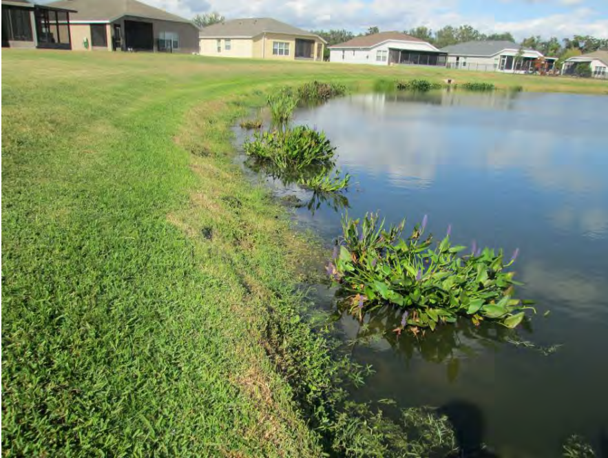
Pond 35 – west bank +/-18” vertical drop, viewing north
