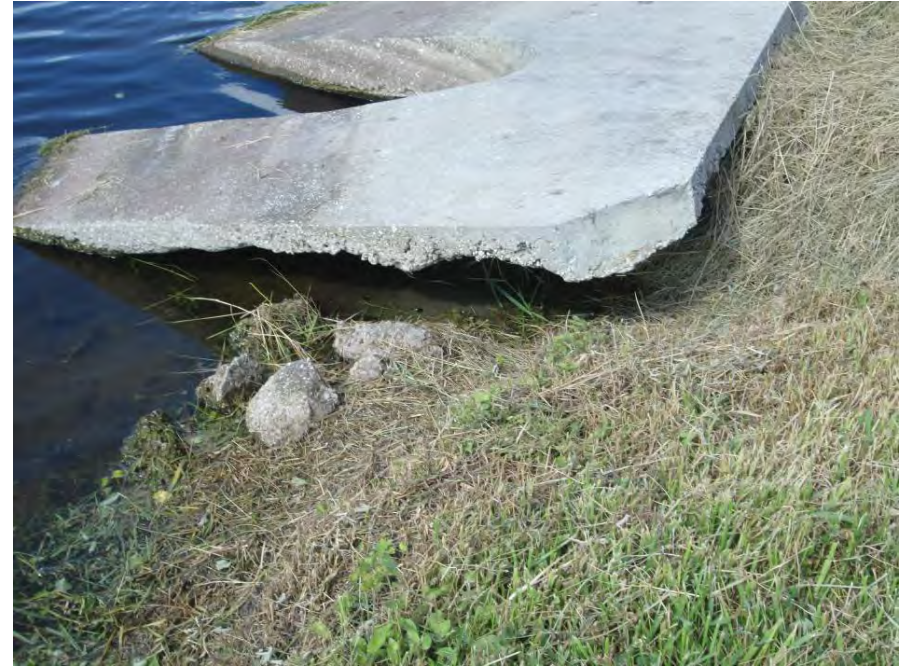
Pond 32 – northeast MES undermined and eroded
