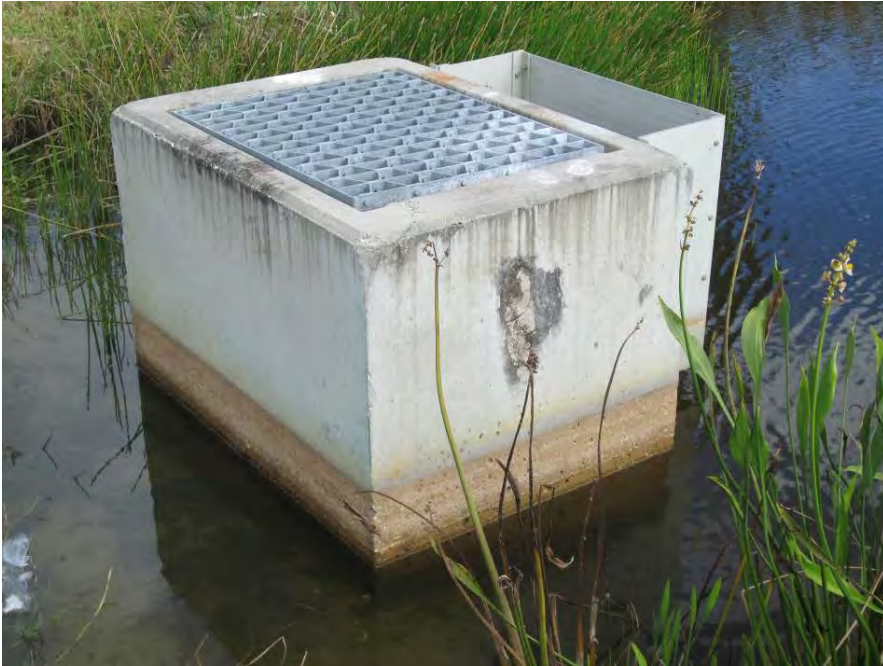
Pond 38 – Control Structure in northeast corner of pond
