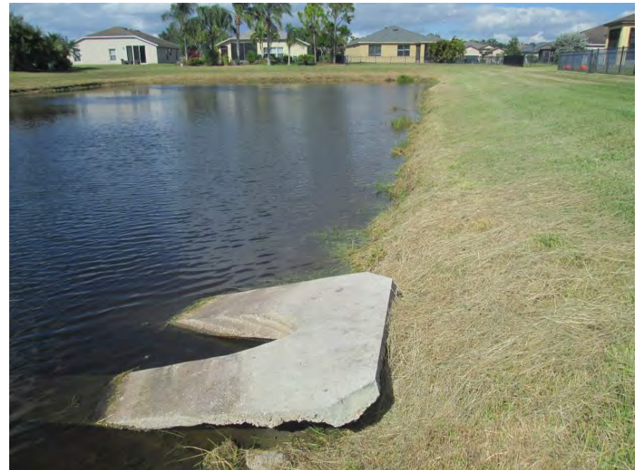
Pond 32 – northeast MES undermined and eroded
