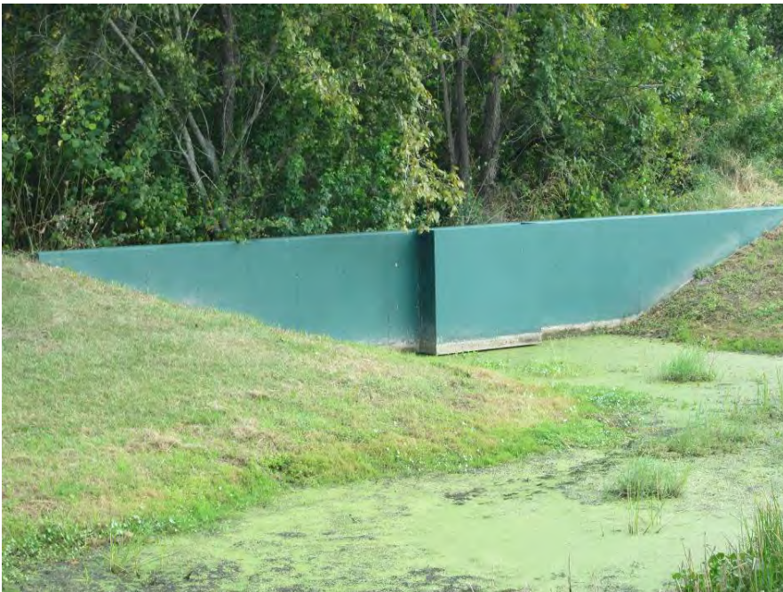
Pond 37 – Outfall weir on northeast portion of pond
