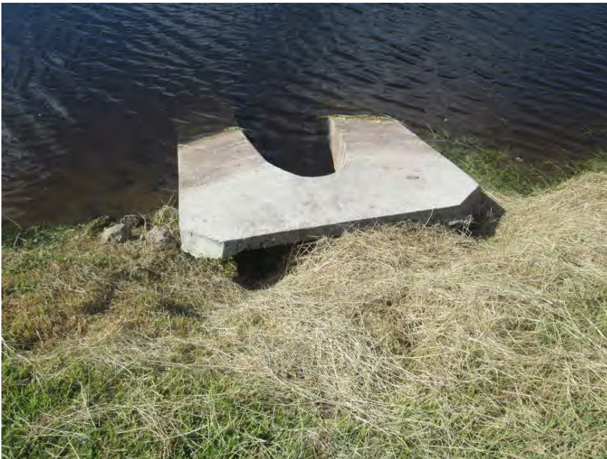
Pond 32 – northeast MES undermined and eroded
