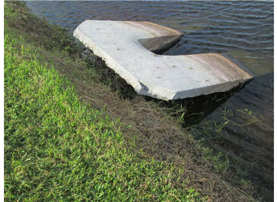
Pond 17 - Undermined & eroded MES on west bank
