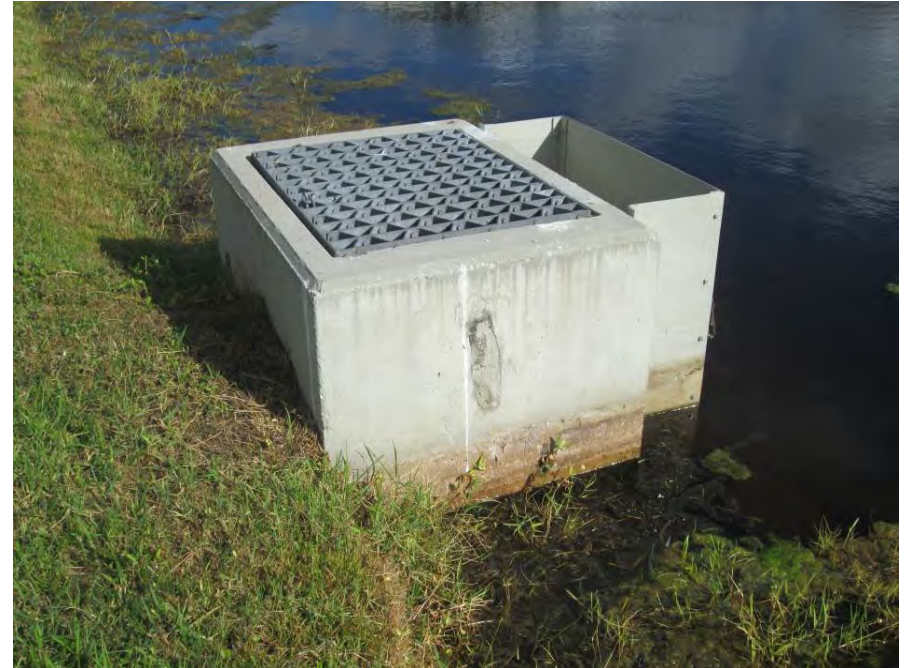
Pond 40 – Control Structure on north bank
